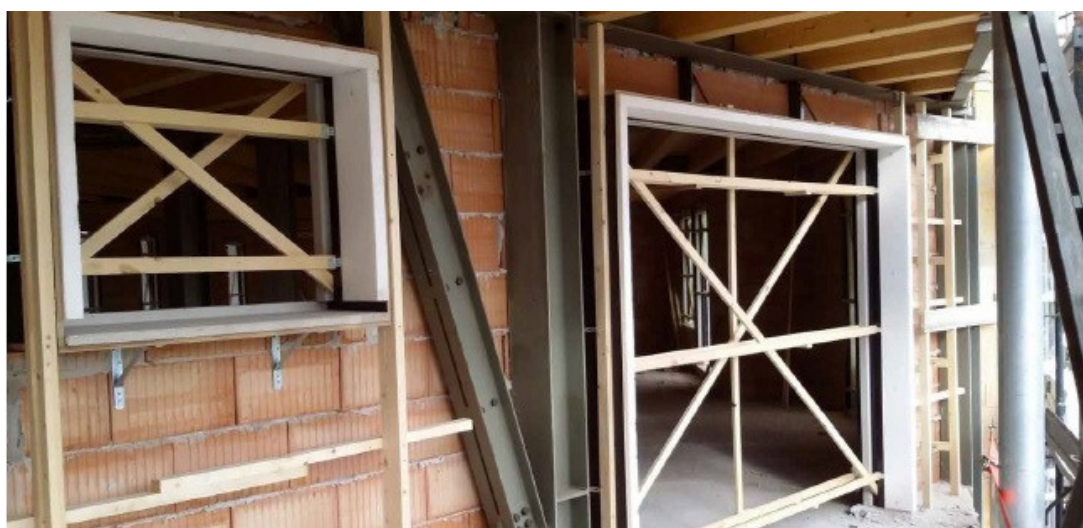
Installation of monobloc basic frame with EPS shoulders supplied by Senini
