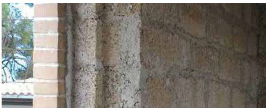
Shaping of the Blocco Ambiente® for housing the basic frame made on site
