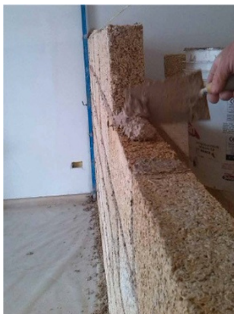
Installation spreading a layer of bedding mortar
