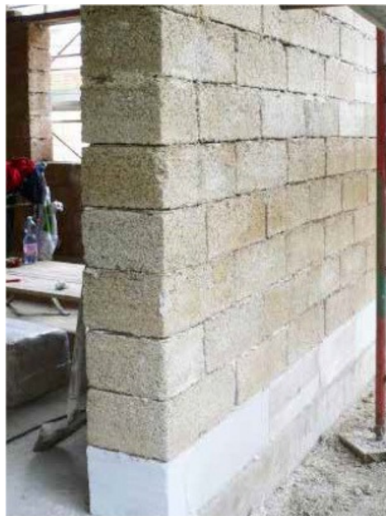
Insulation of the first course with cellular glass
