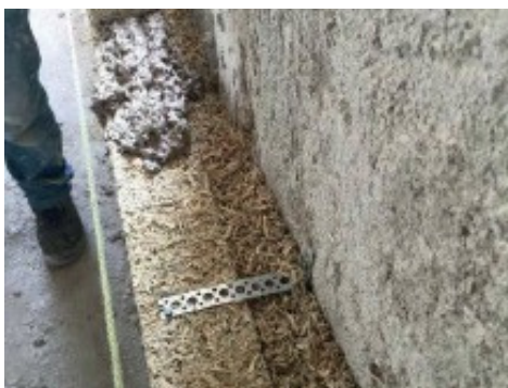
Counterwall of Blocco Ambiente ® with a cavity filled with Bio Beton ®200 Pronto
