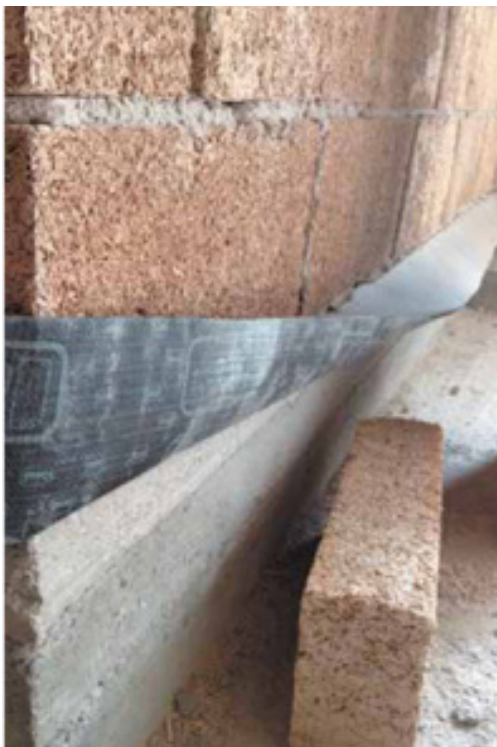
Insulation of the first course with waterproof membrane
