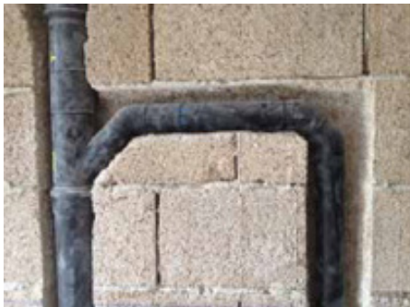
Grooves on Blocco Ambiente® for sanitary system
