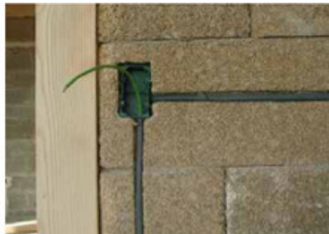
Grooves on Blocco Ambiente® for electrical system
