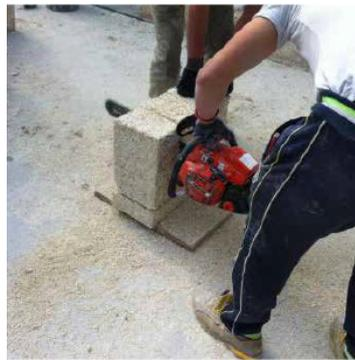
*Blocco Ambiente*® cutting with electric chain saw
