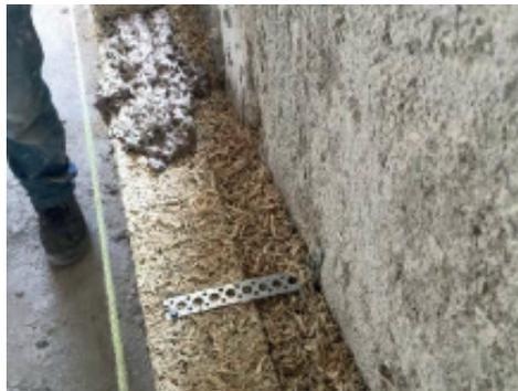
*Counterwall of Blocco Ambiente<sup>®</sup> with a cavity filled with Bio Beton<sup>®200 Pronto</sup>*
