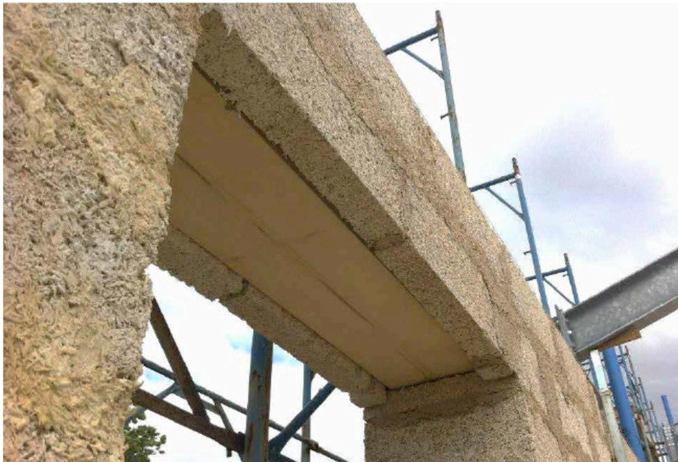
*Installation of a dried wood lintel on a wall in Blocco Ambiente® including the correction for thermal bridges*
