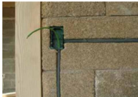
Grooves on *Blocco Ambiente*<sup>®</sup> for electrical system
