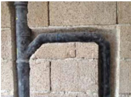
Grooves on *Blocco Ambiente*<sup>®</sup> for sanitary system
