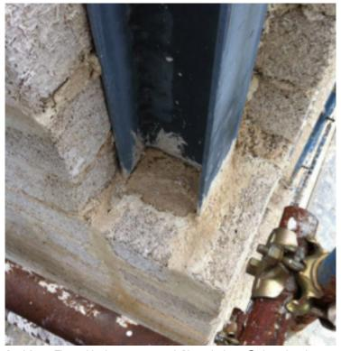
Steel frame:Thermal bridge correction with Blocco Ambiente  $^{\circledR}$  shaped at the corner column
