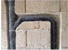
Grooves on Blocco Ambiente® for sanitary system
