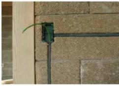
Grooves on Blocco Ambiente® for electrical system
