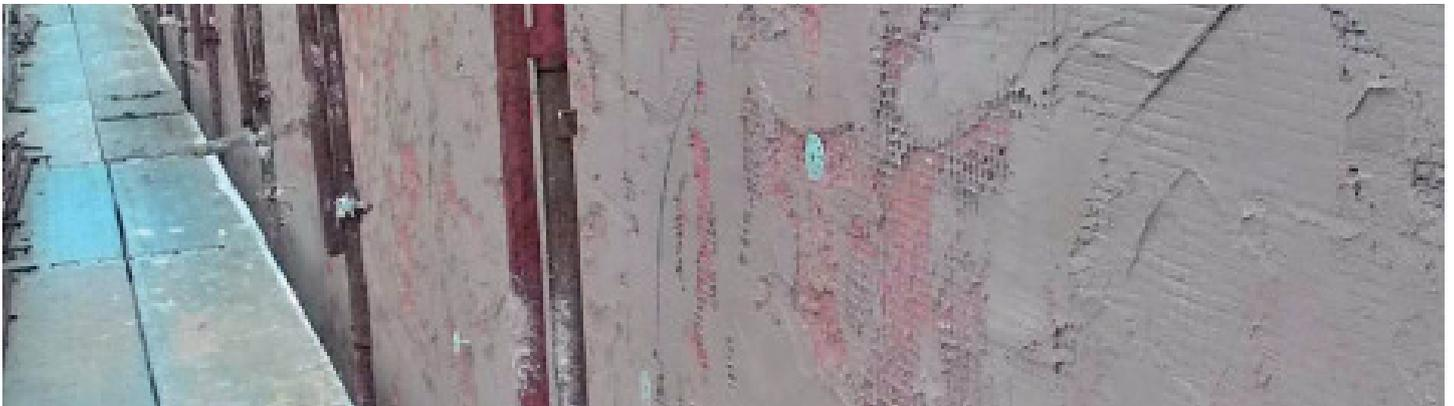
*Application of an overcoat mesh with a first coat of Stabilitura Naturale Traspirante Plus*
