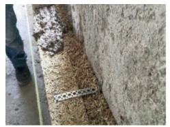
Counterwall of Blocco Ambiente® with a cavity filled with Bio Beton®200 Pronto
