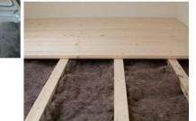
Comfort Insulation (14kg/m³) Thermal Conductivity 0.042 W/m2k
