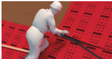
Self-sealing longitudinal overlaps (ADB membrane).
