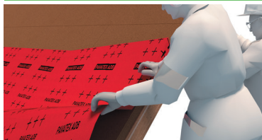
Sealing along the gable ends. PAVATAPE 12 (ADB membrane)
