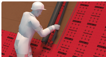
Sealing lateral overlaps with PAVATAPE 12 (ADB membrane).
